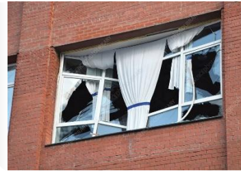
Window damage after ~20m meteor air burst over Chelyabinsk, Russia.
