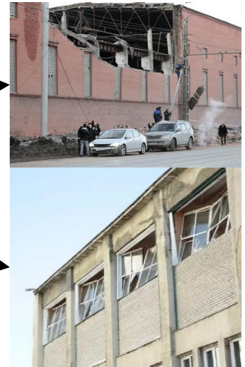
Building and window damage after Chelyabinsk event.
